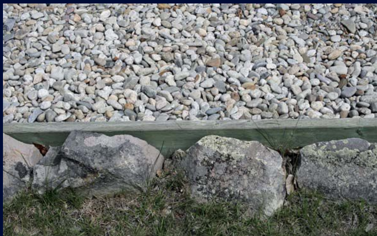
In order keep the drain rock contained, Tabor likes to use treated 2x6s backed by large rocks to maintain their placement.
