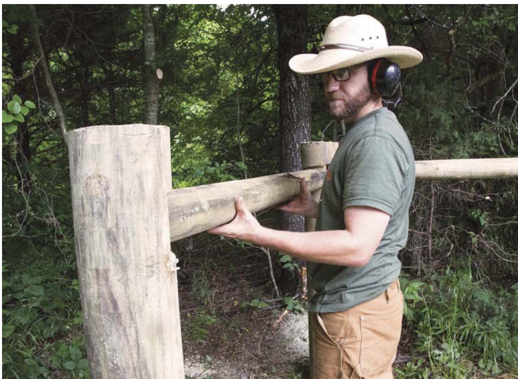
(top) Using a chainsaw, notch the posts so the cross posts sit level. (right) The cross posts give strength to the three-post corner.
