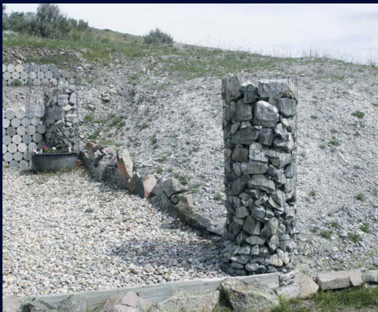
Decorative posts can easily be made by forming a coil of heavy-gauge livestock mesh wire, then filling it with large rocks.
