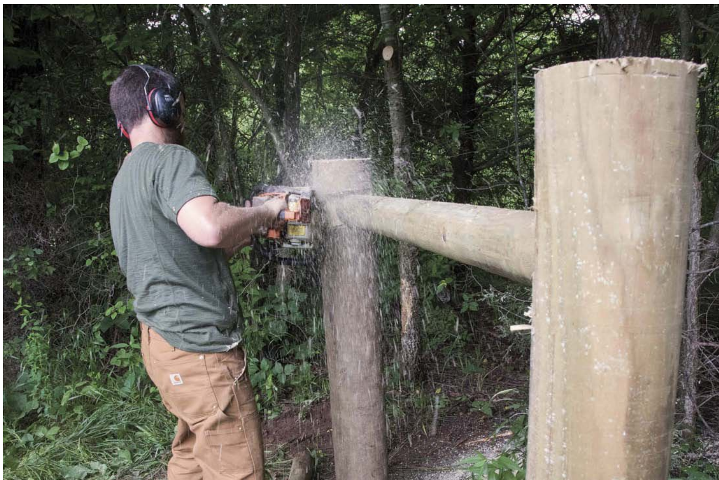
(top) Using a chainsaw, notch the posts so the cross posts sit level. (right) The cross posts give strength to the three-post corner.
